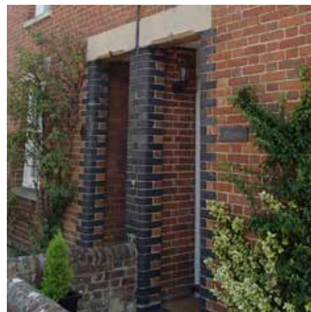
Localised brick detail around doorways
