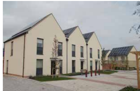
A shared surface street - NW Bicester
