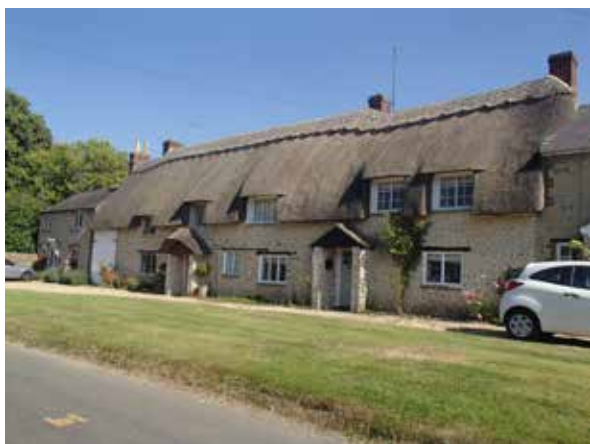
Limestone villages of the south- Islip (top) and Fringford (bottom)
