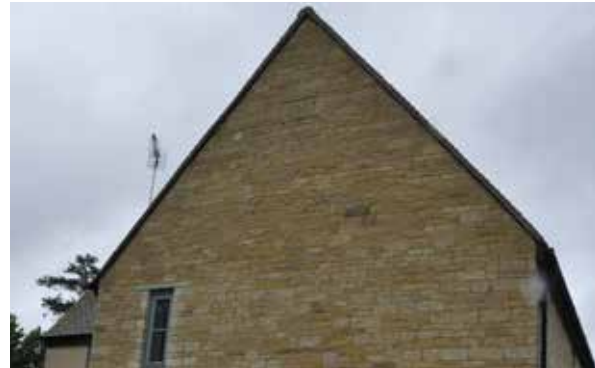
Steeply pitched roof with no overhang, Bletchington
