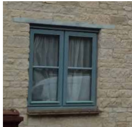
Casement window flush with wall, Bletchingdon
